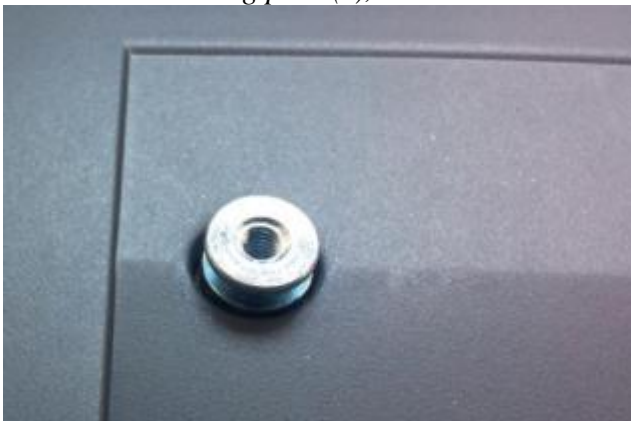
Threaded Mounting point(s), 4mm screw
